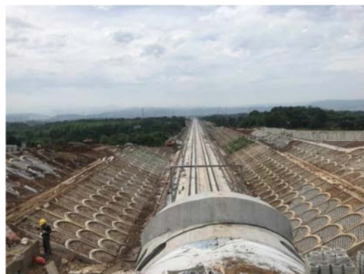
Figure 23. track have been lay on diatomite subgrade.
